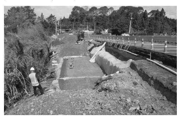
The other AT safety projects that have been constructed along DFH since my last report, include the widening of the intersection of DFH and Bawden Road, the installation of a new righthand turning bay and safety barriers.
